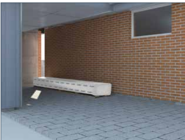
If storing on site for more than 2-3 weeks, the product should be kept under a roof. A maximum of 4 panel or 8 plank pallets can be stored on top of each other.
